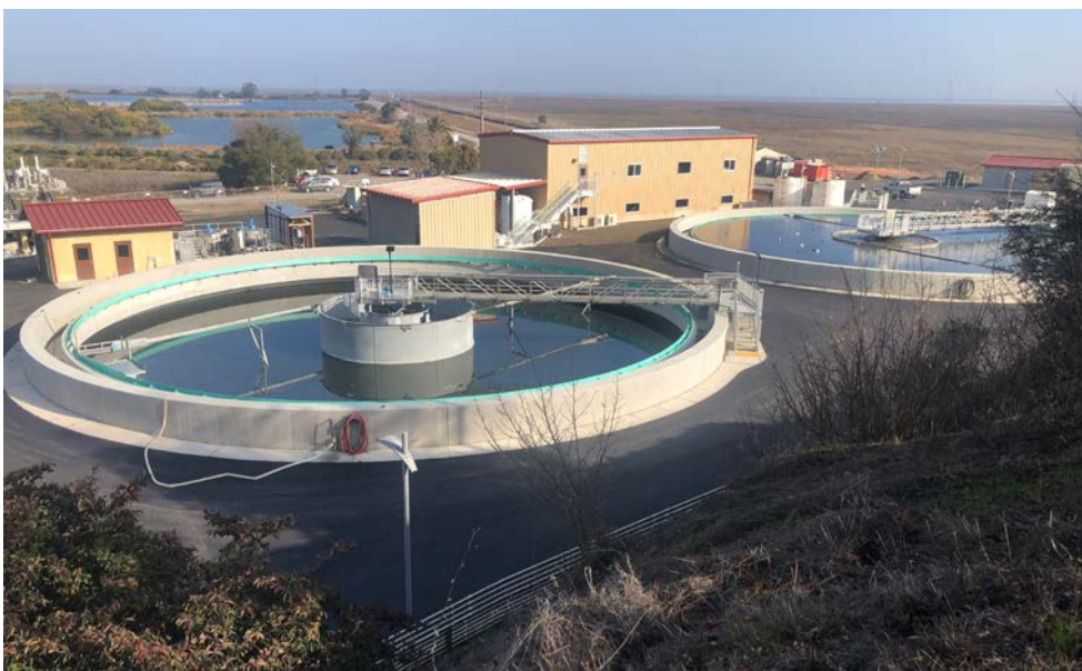
New wastewater clarifiers are part of the recently completed Secondary Treatment Plant Upgrade and Recycled Water Expansion Project.
