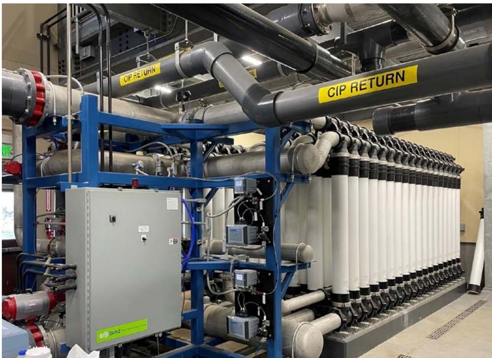
Recycled water membrane filter system
