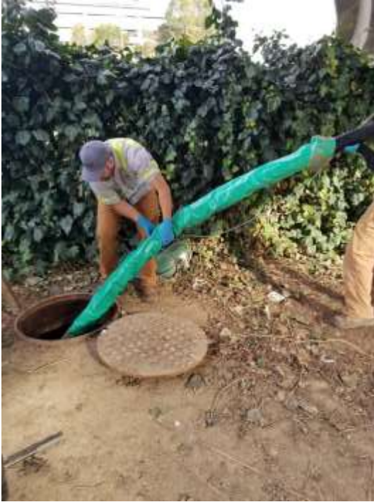
RVSD staff removing plug
