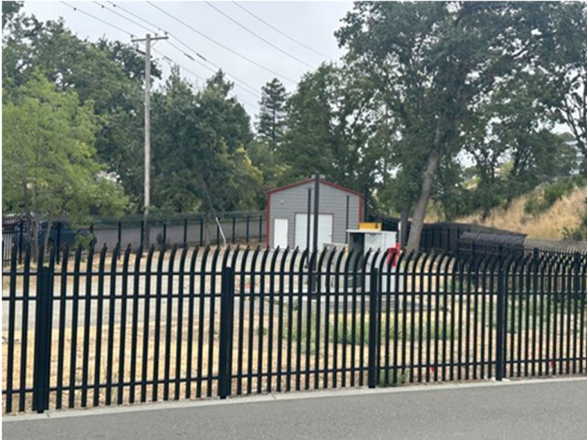
Rafael Meadows Pump Station Improvements
