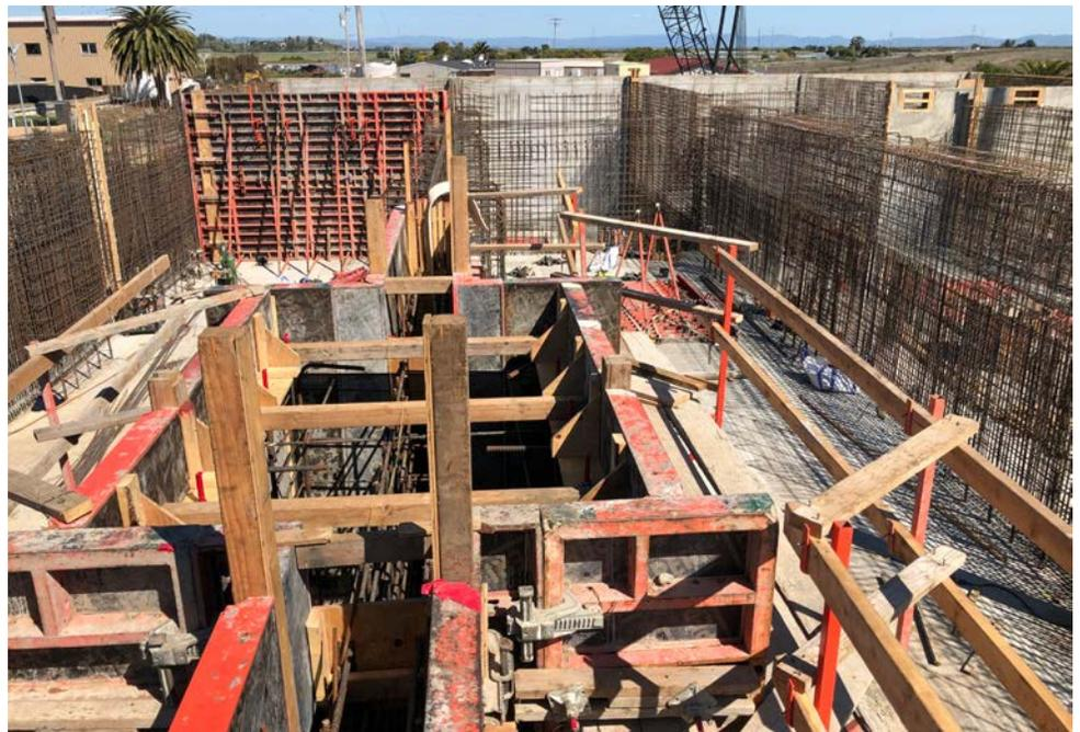
*Aeration basin interior walls formwork and rebar.*
