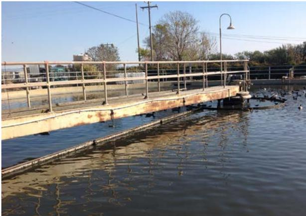
*The Secondary Clarifier is used to remove floating solids and solids that have settled to the bottom. It no longer meets safety standards.*
