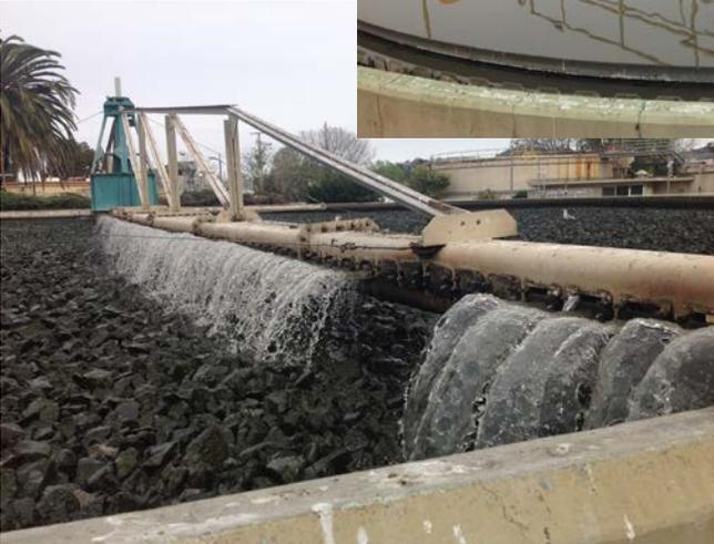
*The trickling filters are part of the biological treatment systems. There is insufficient treatment capacity and it is unable to meet new requirements.*
