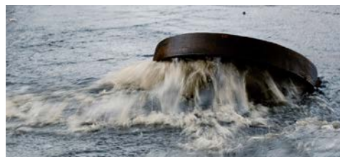
The District must take action to prevent sewer overflows that occur during wet weather events.
