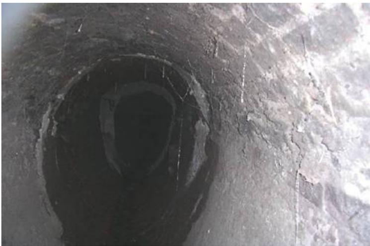
Water can “infiltrate” sewer pipes through leaks in pipe joints and connections or through breaks and cracks.
