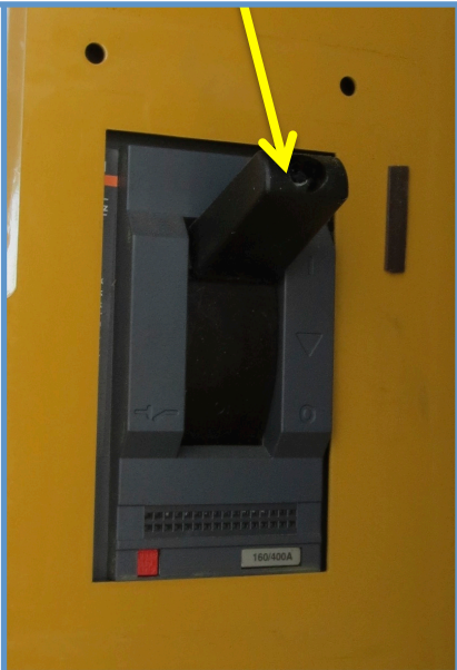
Generator disconnect switch
