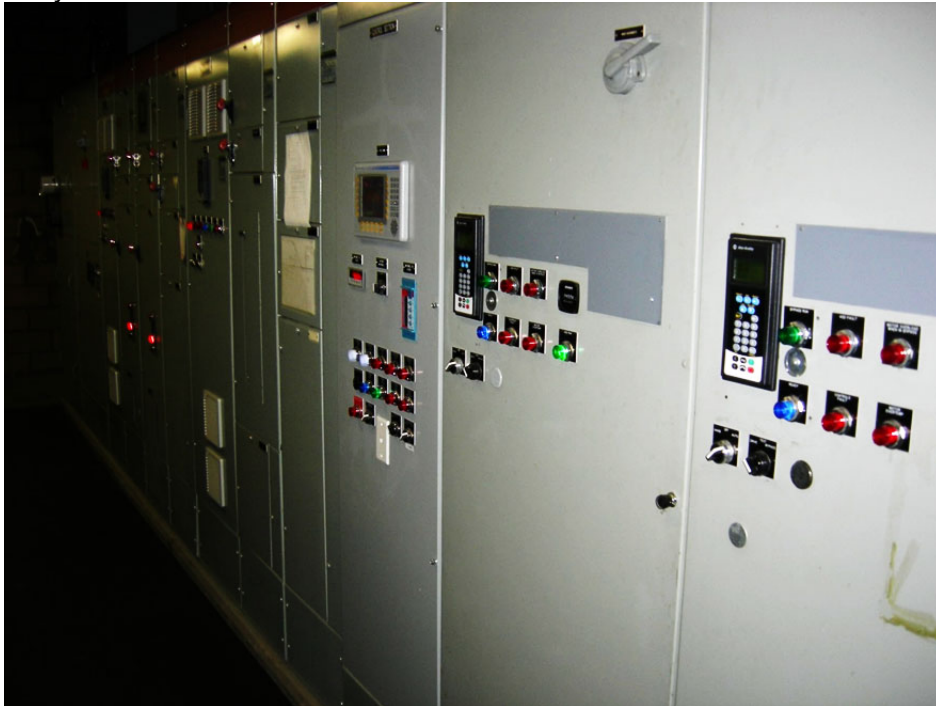
Recycled water treatment facilities
