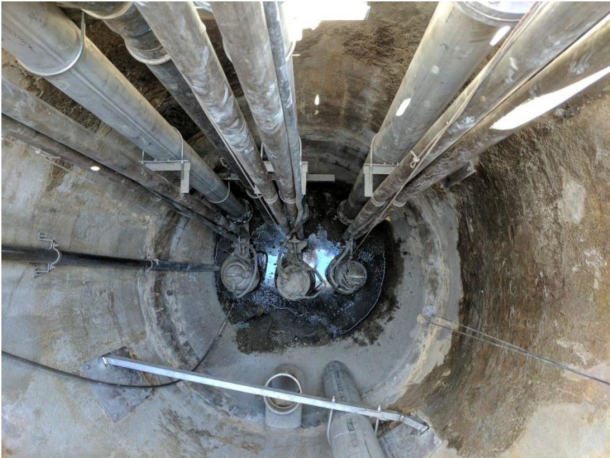
Descanso pump station wet well upgrade project
