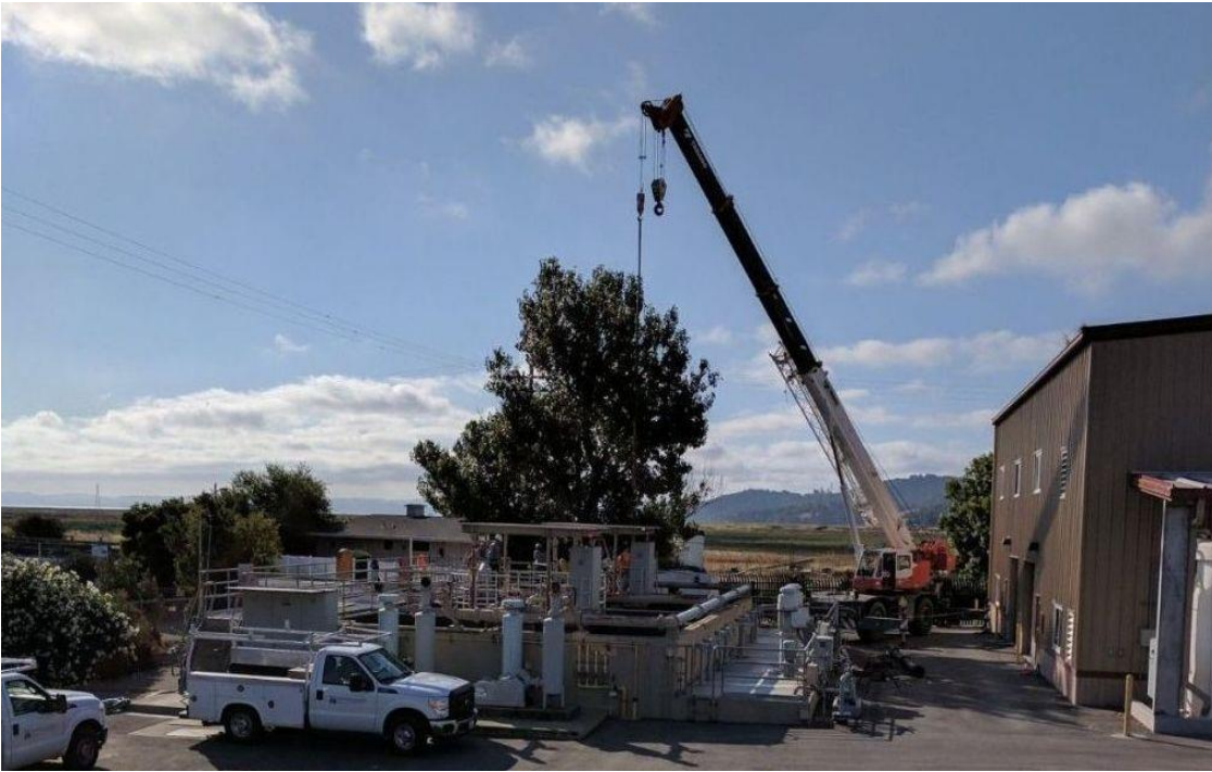
Deep Bed Filter Inlet Valve Replacement Project
