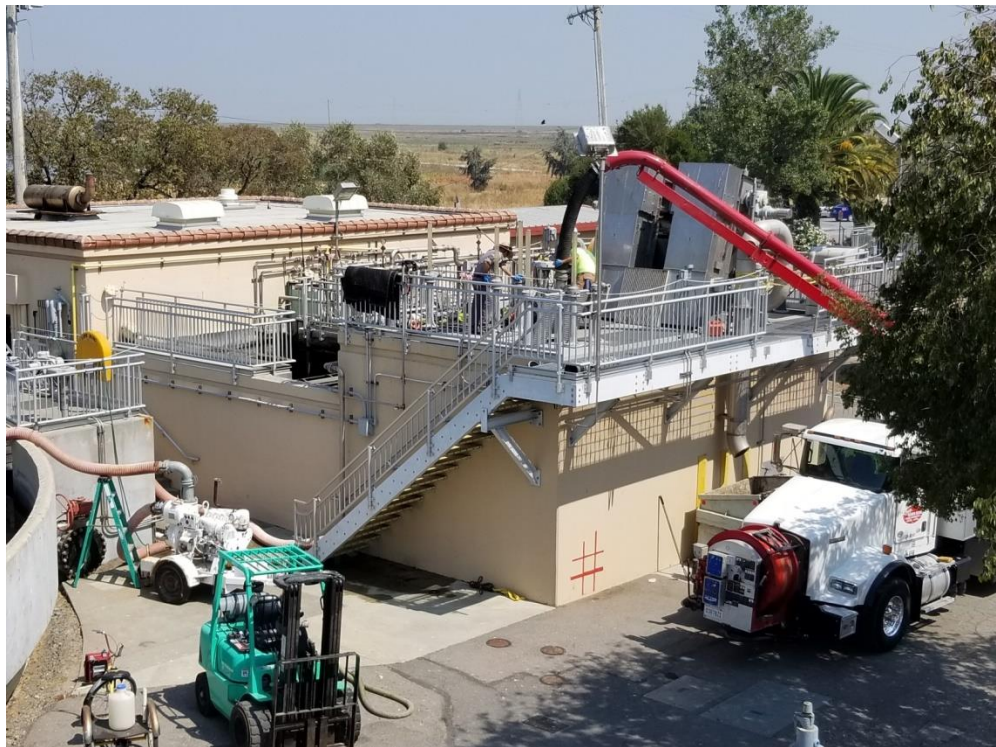
Operations Staff and Sewer Services Contractor Cleaning the Plant Headworks Channels
